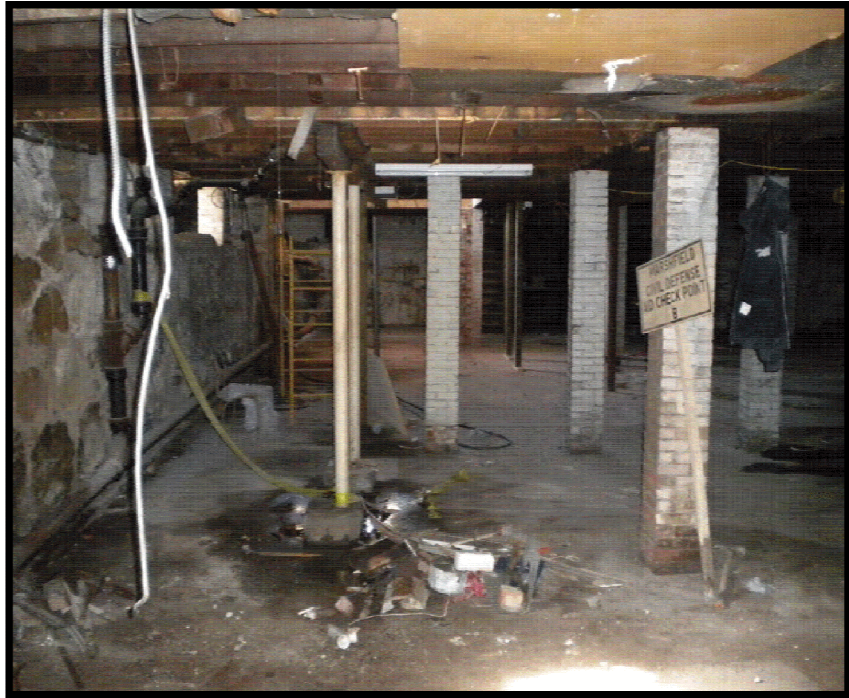
Ground floor demolition in progress.
